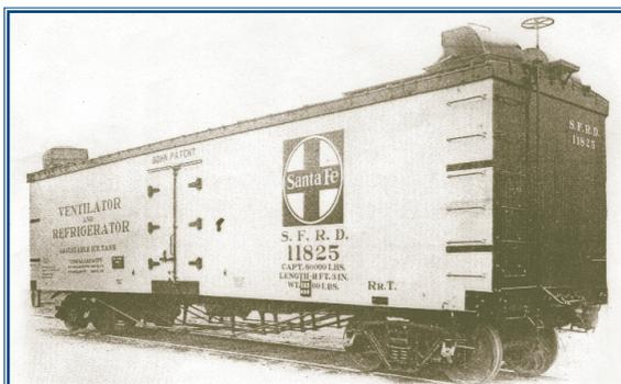
Wooden Refrigerator Car with Collapsible Bulkheads.
