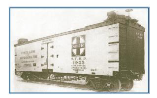
Wooden Refrigerator Car with Collapsible Bulkheads. Capacity, 30 Tons; Weight, 52,000 lbs.; Length between Bulkheads, 33 ft. 2-1/4 in.; Inside Width, 8 ft. 2-3/4 in. Builder, American Car & Foundry Co.
